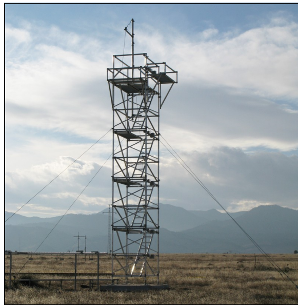
A NEON prototype tower at Colorado's Table Mountain. Similar towers, outfitted with environmental monitoring equipment, will be erected at sites in NEON's 20 eco-domains throughout the United States.
