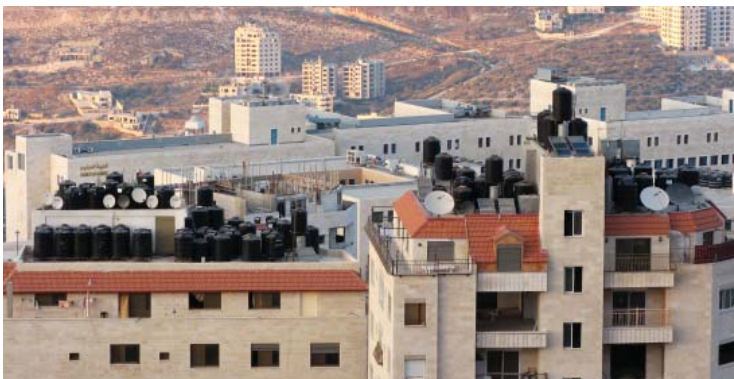
Due to the water shortage in Nablus, the city can only provide drinking water every few days. Residents have to stock up on water by storing it in large tanks on their roofs to use during the in-between days.
