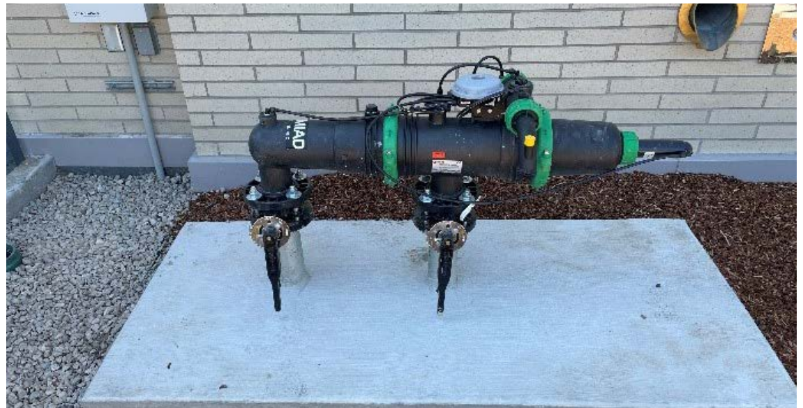
Secondary filter for drip areas
