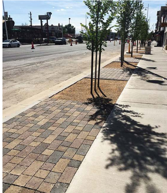
Portions of a streetscape are paved for walkability
