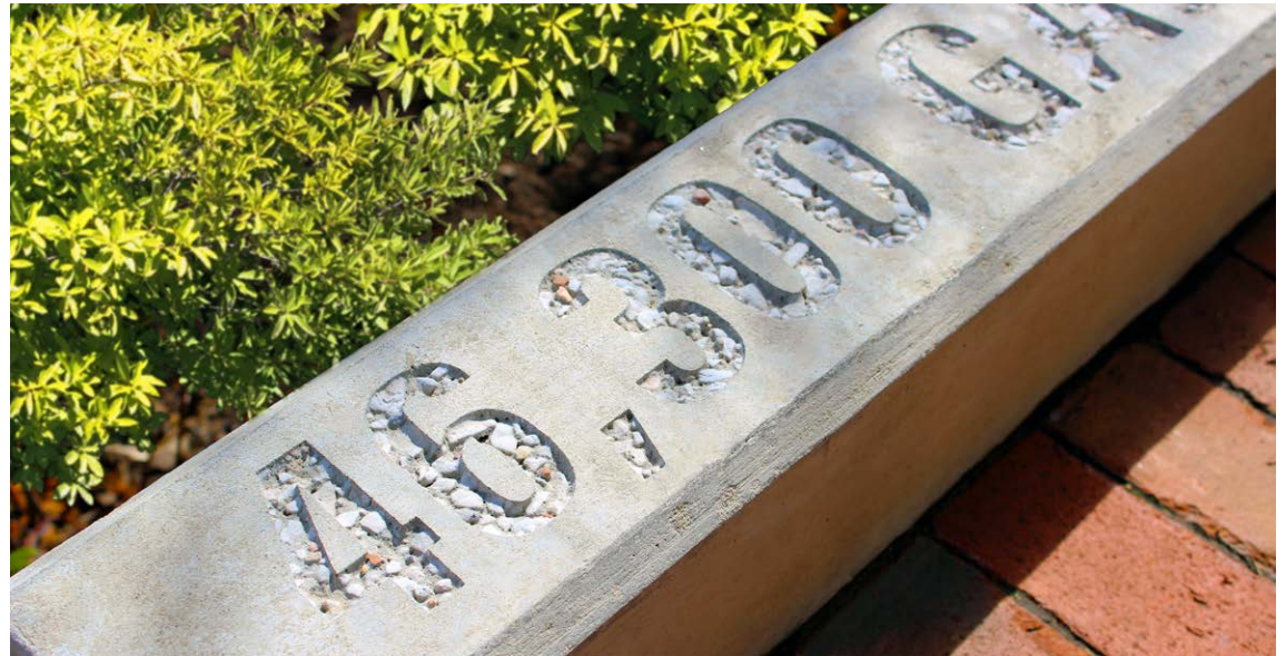
Water savings sandblasted into a concrete curb
