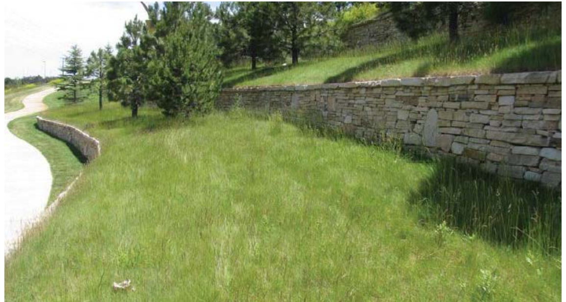
Fine fescue grassland with retaining walls
