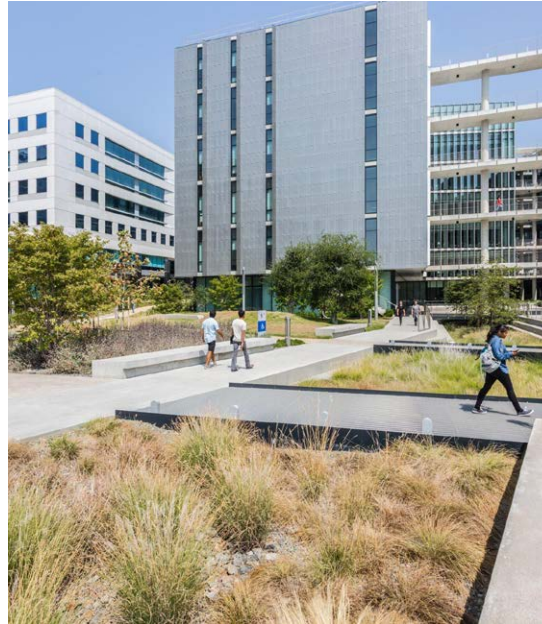
Stormwater treatment within a landscape approach
