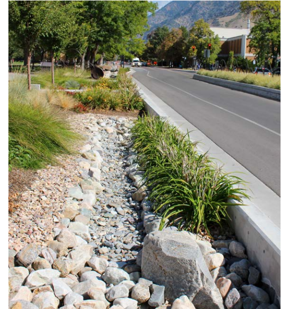
Stormwater treatment within a streetscape design
