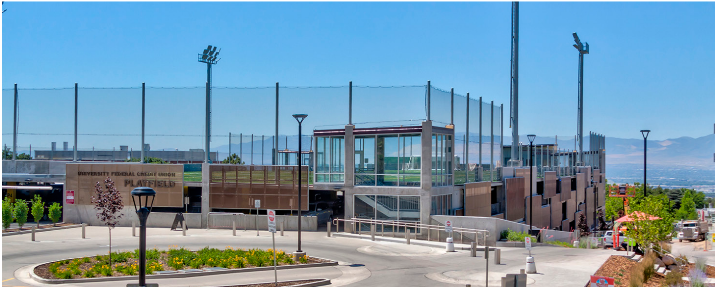
University of Utah Business Loop Parking Structure built across a site with significant grade change
