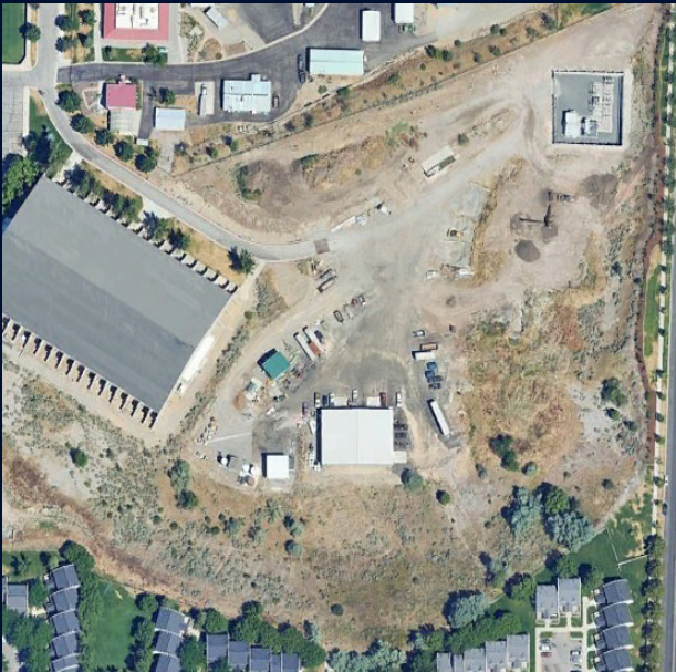
Coal Yard Area
