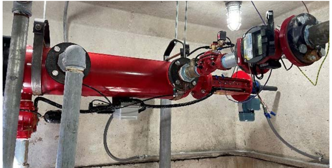
Self-flushing filtration system
