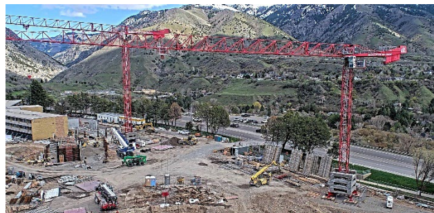
Figure 2. South Campus Construction
