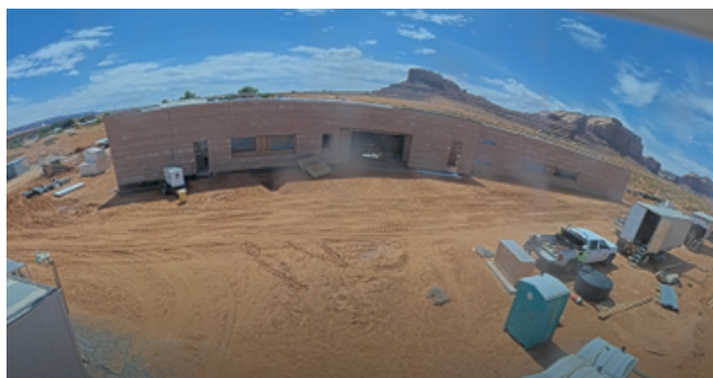
Figure 1. Monument Valley Academic Building
